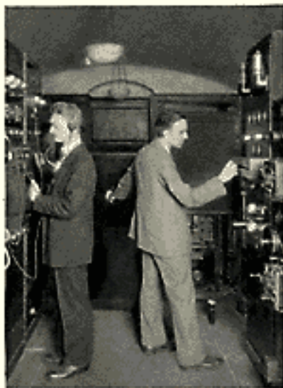
The nerve center of the photoelectric eyes of the television equipment installed at Washington. G. R. Keith and J. G. Knapp of the Laboratories manipulate the controls at the amplifiers which transmit the scene to New York
